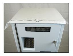
2. Center hole saw on template and score Sentinel. When finished, remove and discard template.
