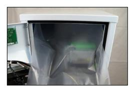
4. Use power drill (not provided) and hole saw to drill hole through score mark.
