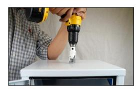
5. Clear area of any shavings, then use alcohol wipes to prepare surface for installation.
